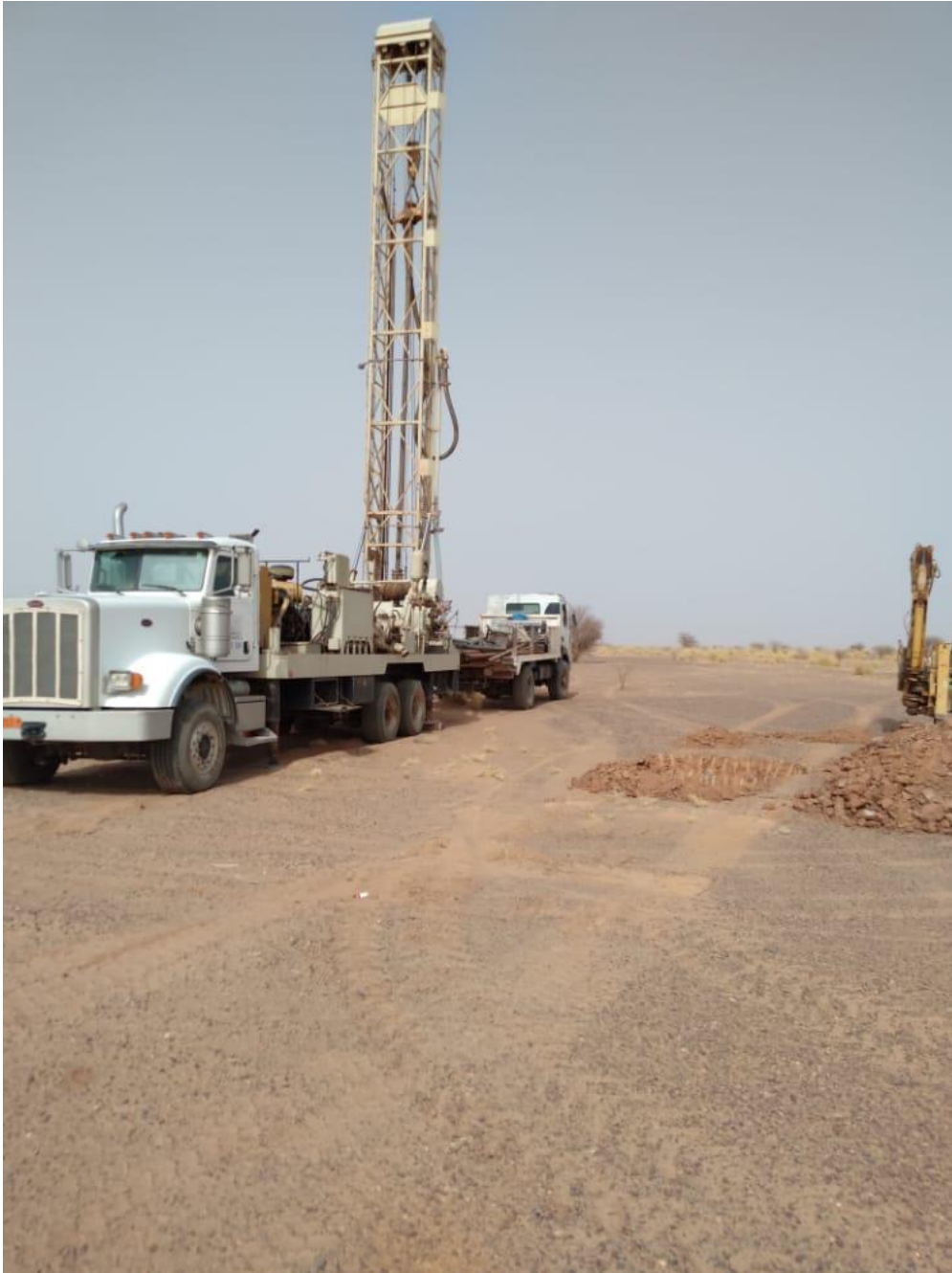
Figure: ESAFOR drilling at Miriam in May 2021
